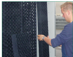
Easily removable combined inlet shields
