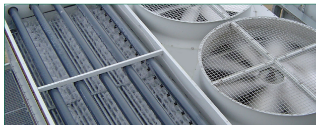
Full access to spray distribution and top of coil during operation
