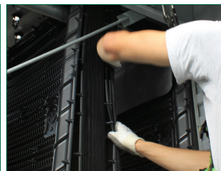
Patented BACross II fill for easy inspection and cleaning
